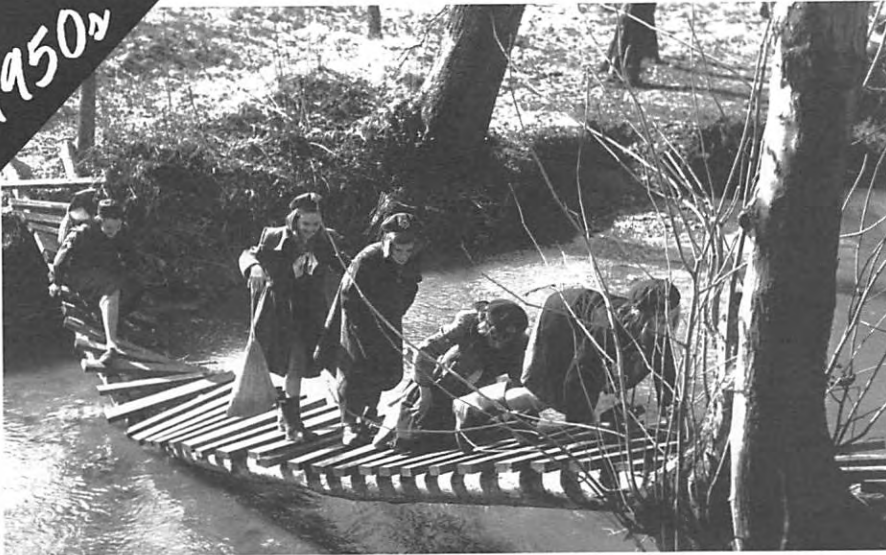
Bridge crossing Pimmit Run – c. 1952-53
