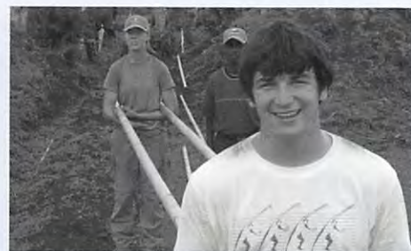
Trevor Lewis '06 carrying water-pipes
