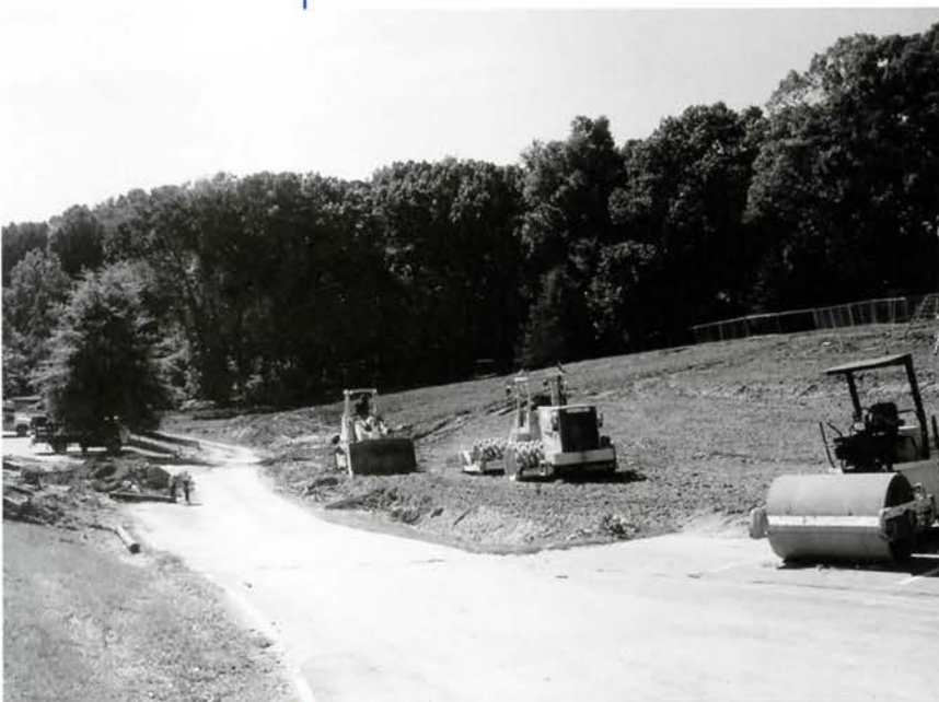
Bulldozers flatten out land.
